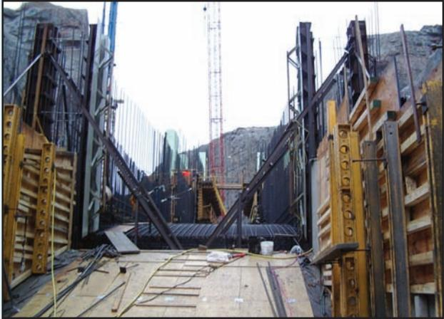
1. Clean all previously used formwork using mineral spirits, acetone or denatured alcohol prior to the application of the form retarder. This step will help the process but is not absolutely required.
