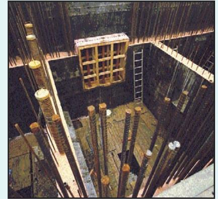
4. After the concrete has reached sufficient strength, the forms are removed. The treated retarder matrix should be removed within 72 hours for proper control of the matrix being removed. Generally with high-pressure water using 1,500-2,000 psi at a rate of 4-6 gallons per minute flow yielding 500-600 sq.ft. / Hour. When employing sand either dry or wet it is important not to damage any coatings that may be used on the reinforcement. Most times water is best suited for removal.
